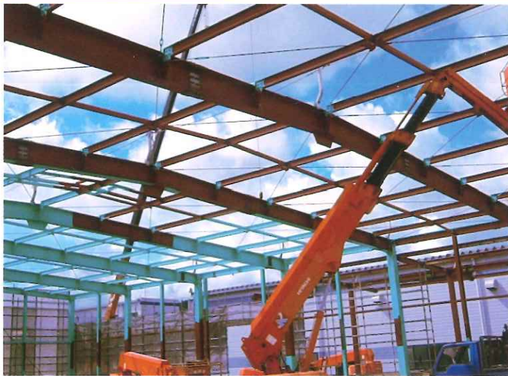
工場新築工事
