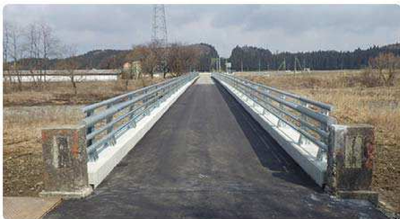
(赤沢橋橋梁修繕工事)
