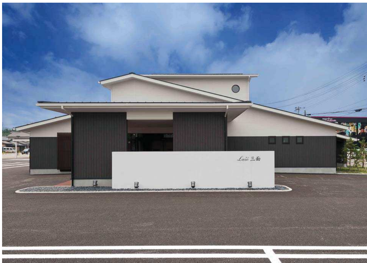
(ラソ三面新築工事)
